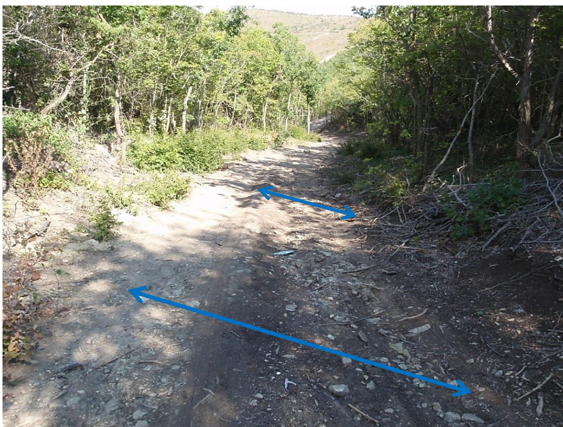
Photograph 10 Access track to drill pad 3 (facing downhill) (blue arrow denotes suggested location of grips)
