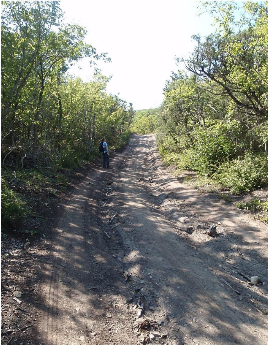
Photograph 11 Soil erosion on Permanent Access Track
