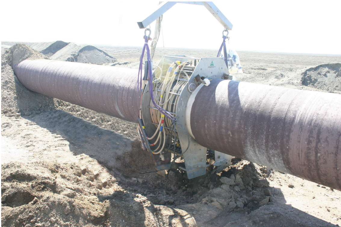
Figure 5.16 Application of Field Joint Coating
