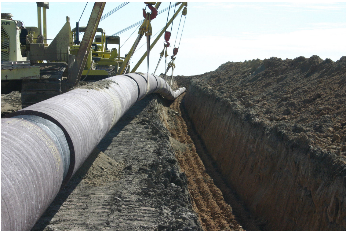
Figure 5.17 Pipe Lowering into Trench
