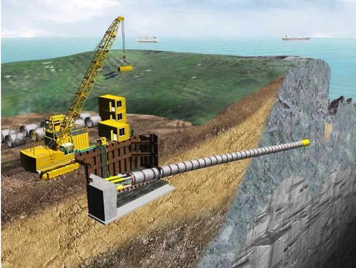
Figure 5.22 Typical Microtunnel Construction
